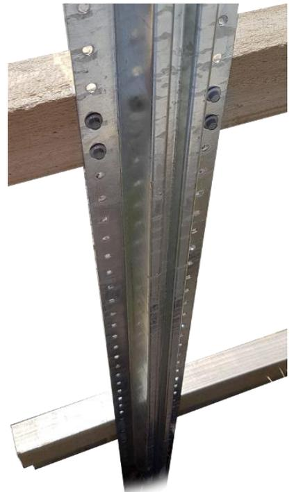
**8.** Place the bottom rail on top of the plinth block and attach to the post using the holes provided.
