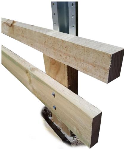
**7.** Next fix the plinth to the plinth block with the top of plinth set to the mark on the block.
